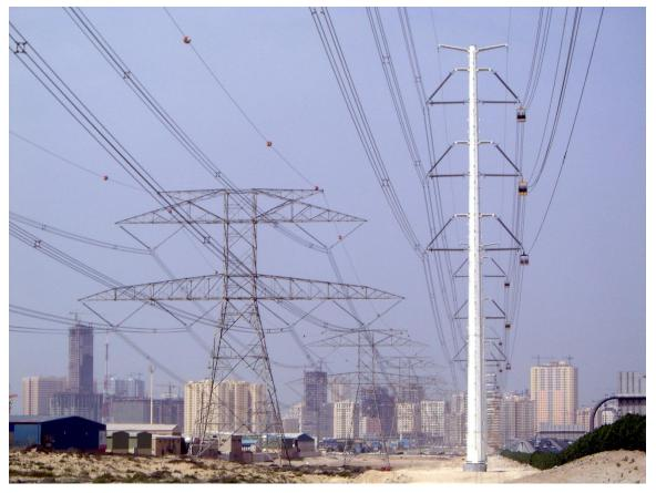
Comparison of standard and compact line design 2 x quadruple bundle
